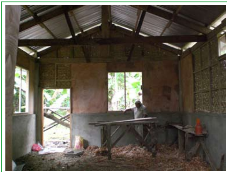
Interior view from the entranceway
