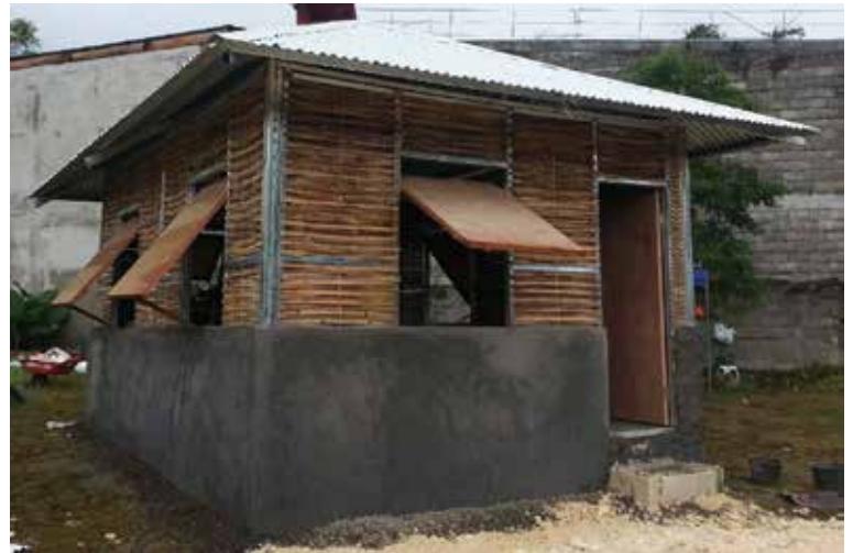
The core shelter model house built by Habitat for Humanity in Tagbilaran City, Bohol. The approximate cost of this house is $2000 CAD.
